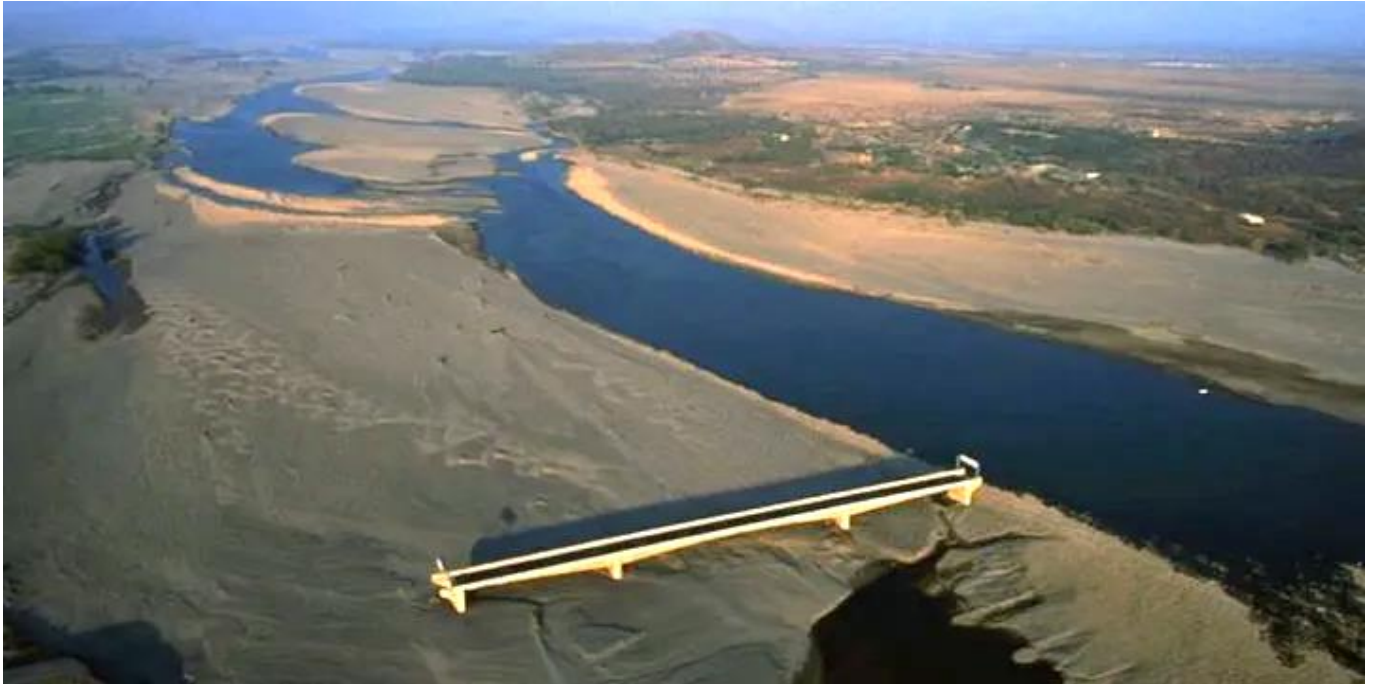
The Choluteca Bridge, Honduras
